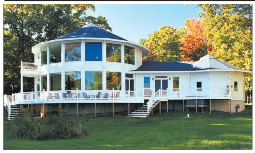
This is a passive solar house with large windows along the southfacing side. The interior has an open floor plan to allow the warm air to freely circulate.
